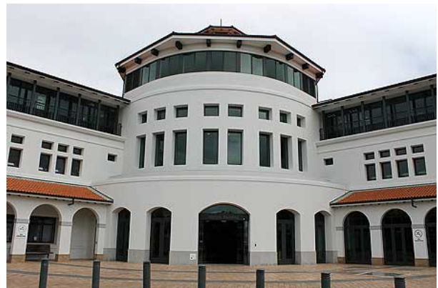
The Atrium Building at Albany
