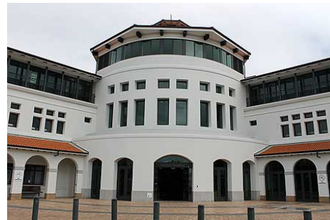
The Atrium Building, Albany campus
