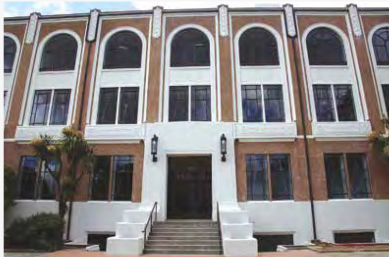
Sir Geoffrey Peren building following the completion of the renovation
