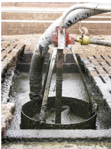
Figure 1 The vertical effluent stirrer.
