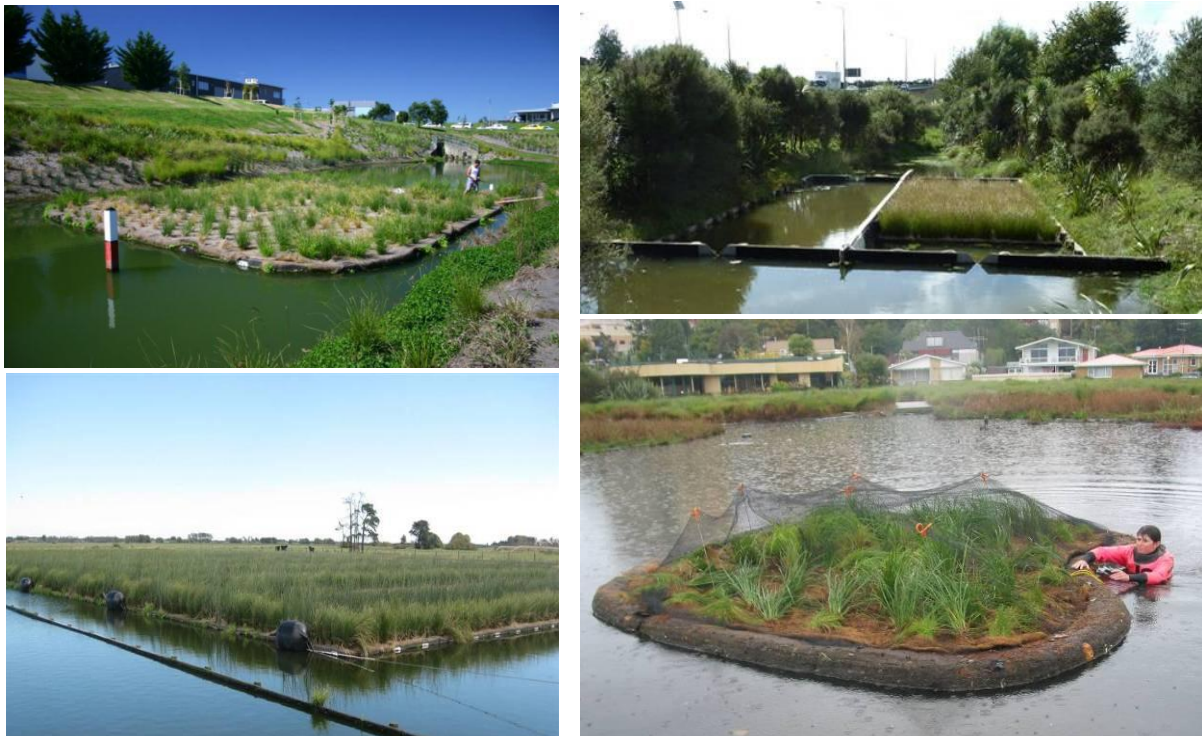
Figure 10. Some New Zealand examples of FTW applications being tested for (clockwise from top left) treatment of urban stormwater (North Shore, Auckland) and road run-off (Northern Motorway, Auckland), lake water quality enhancement (Lake Rotoroa, Hamilton), and treatment of wastewaters (Shannon WTP, Manawatu)
