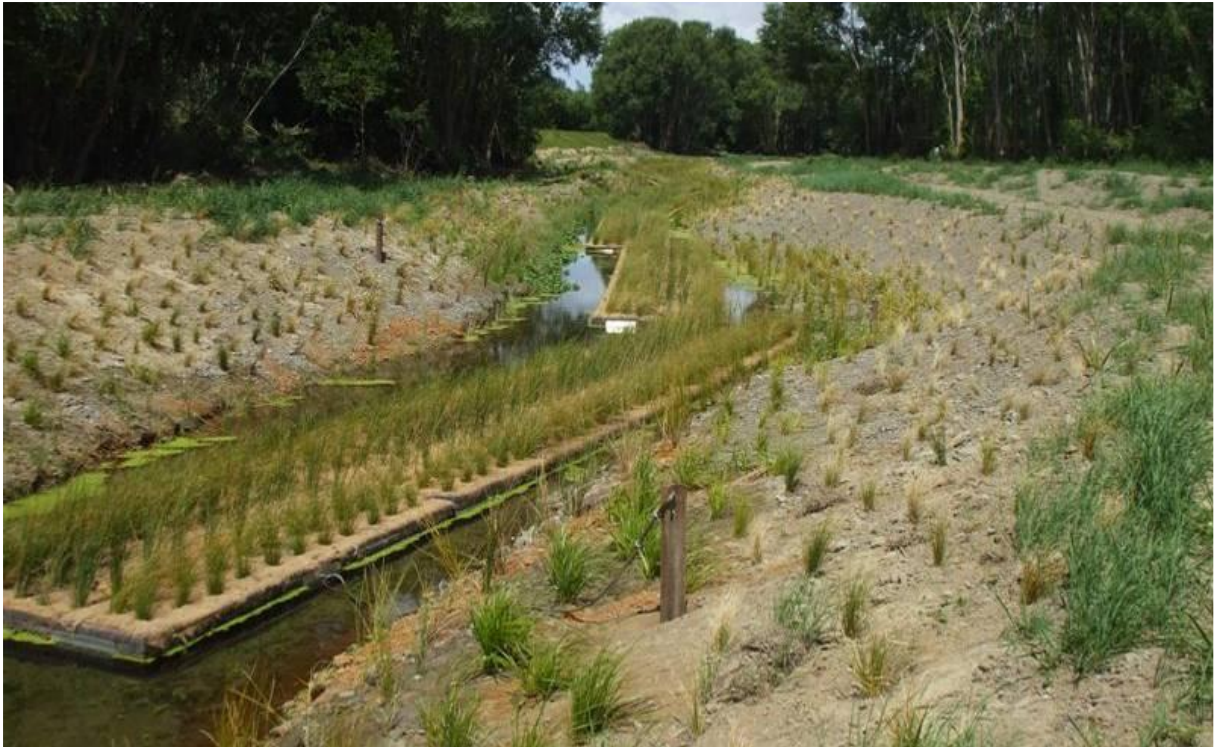
Figure 9. Trial application of FTW for treatment of agricultural drain-flows into the Tukipo River, Hawkes Bay Regional Council.
