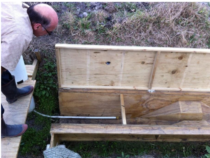
Figure 10: Tatuanui farm (lower site) flume box. Note that the front of the flume box is open and the surface drain is blocked to allow all water from the surface drain to enter flume box.
