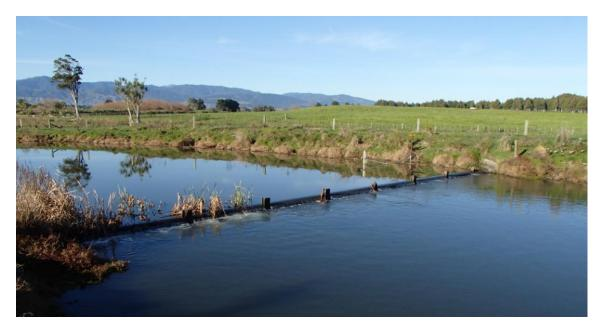
**Photo 3:** Weir along the Hokio Stream which impedes fish migration from the ocean to Lake Horowhenua.
