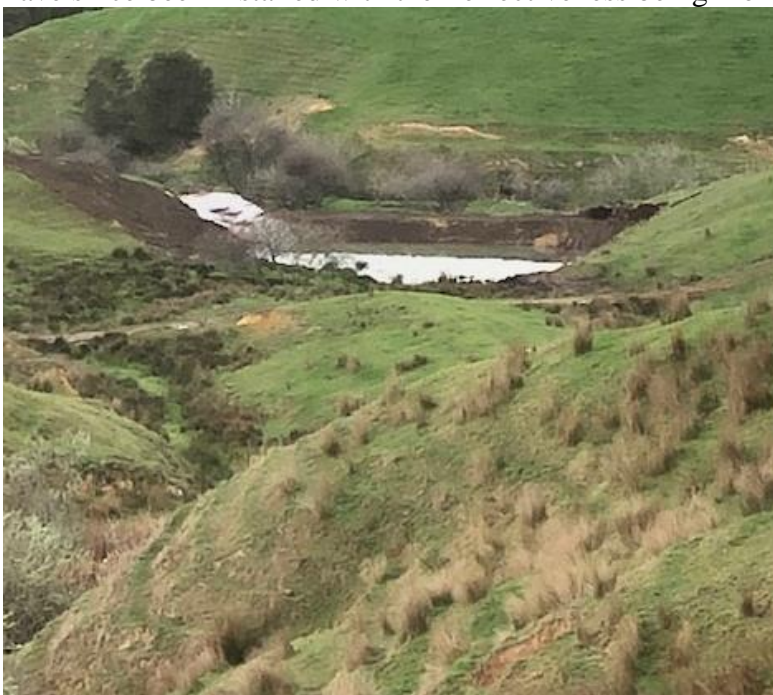
Figure 8: Example of sediment trap.
