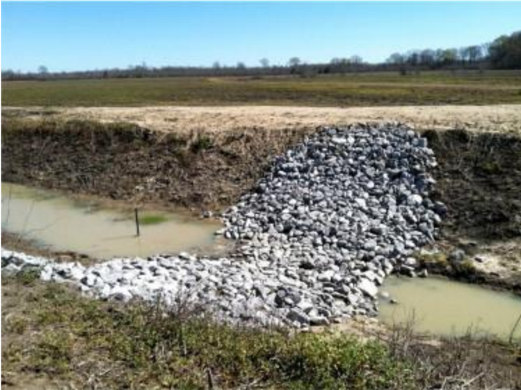
Figure 13: A low-grade weir in Mississippi (from Prince Czarnecki et al 2014).
