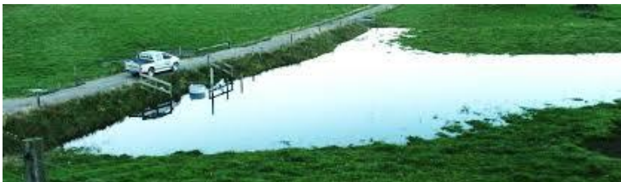
Figure 16: Ponded drainage temporarily impounded behind a detainment bund created from a causeway road (from Clarke et al. 2013).
