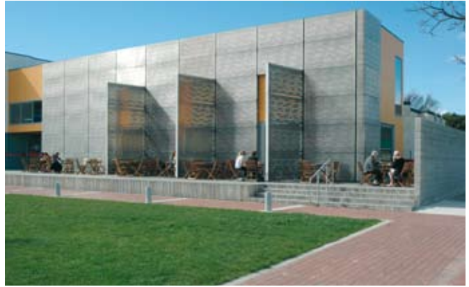
This page: Image and detail of Rainscreen (2007) facade, a collaboration with Athfield Architects and Fraser Engineering. The New Dowse, Lower Hutt.
